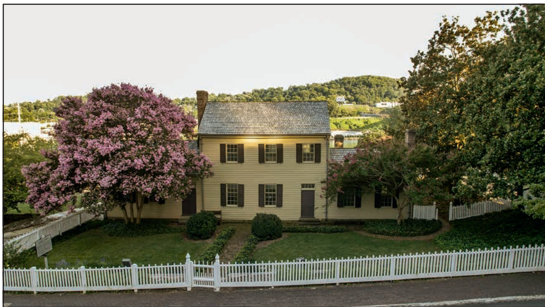
Blount Mansion, present-day photograph of façade.
