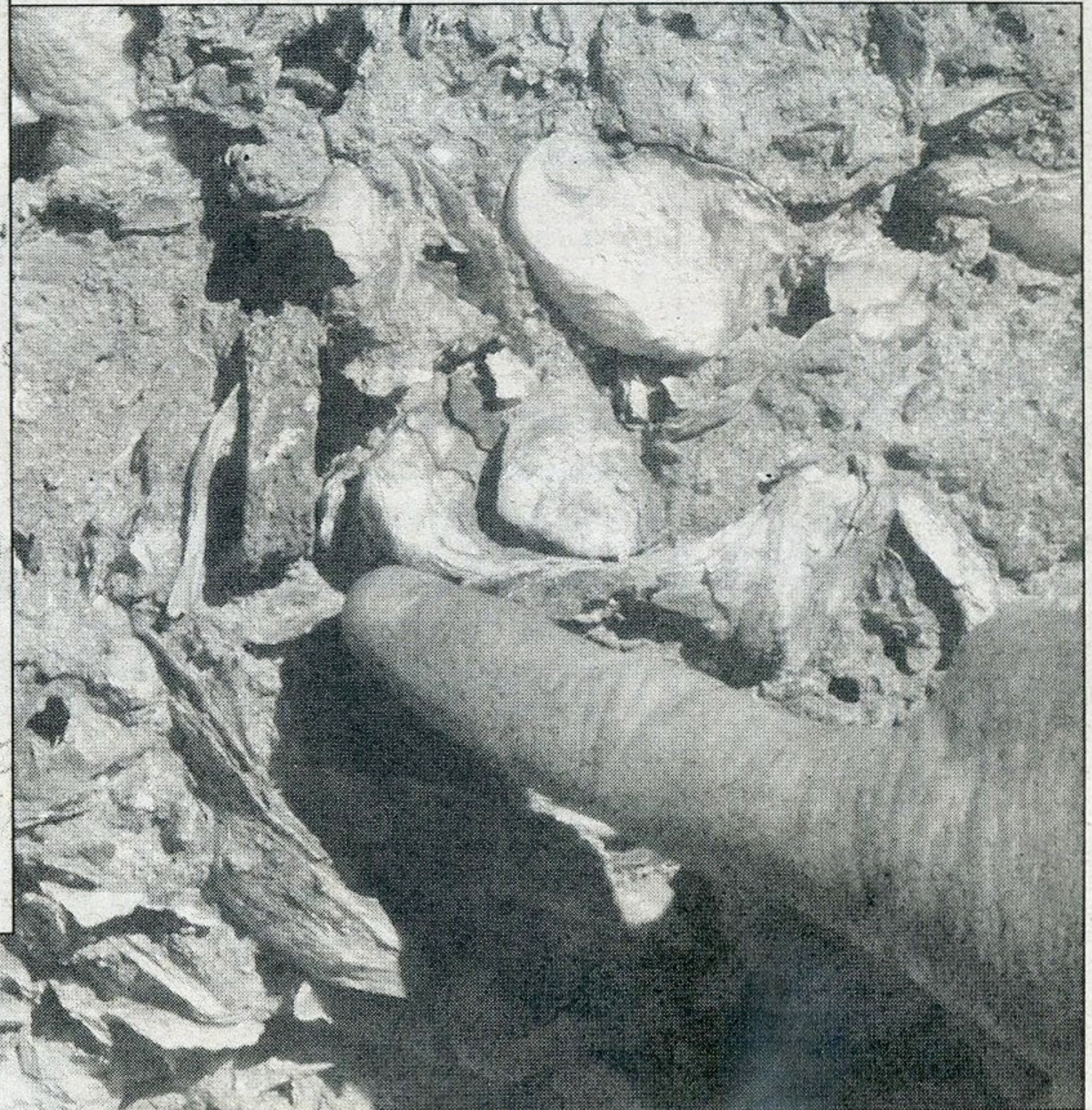
Above: Jim Bitler of the Ossabaw Foundation points to a prehistoric piece of Native American pottery embedded in the tabby wall of one of the slave cabins. Builders typically used ancient Native American shell middens (large piles mostly comprising the debris of consumed shellfish) to make tabby for buildings
